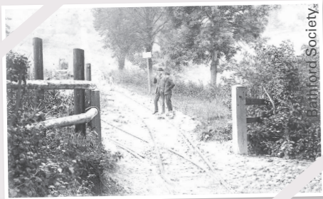
Tramway at nearby Monkton Farleigh c. 1886. The tramway was used to transport stone extracted from mines in the area
