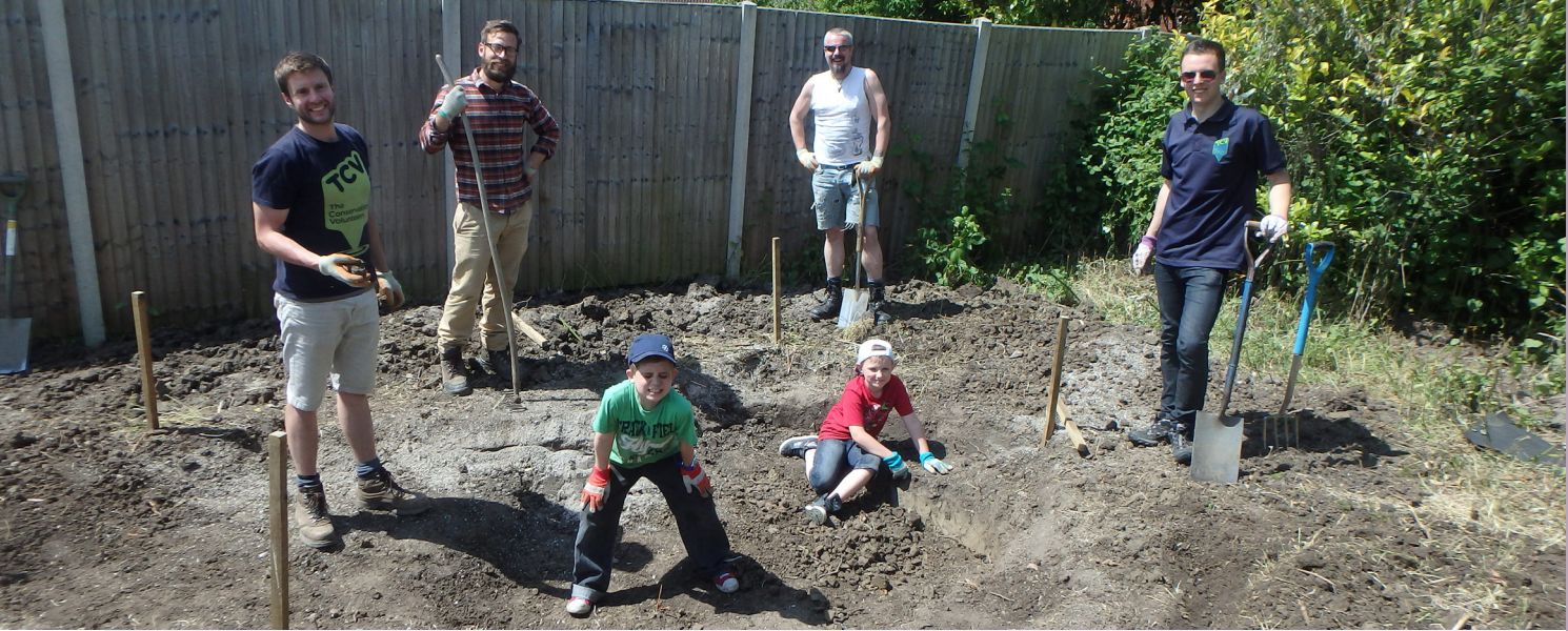
Digging a hole for the new pond at Coleridge Road Allotment
